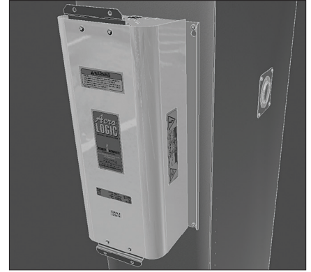
Attach unit using the face mounting bracket and self-drilling screws.
